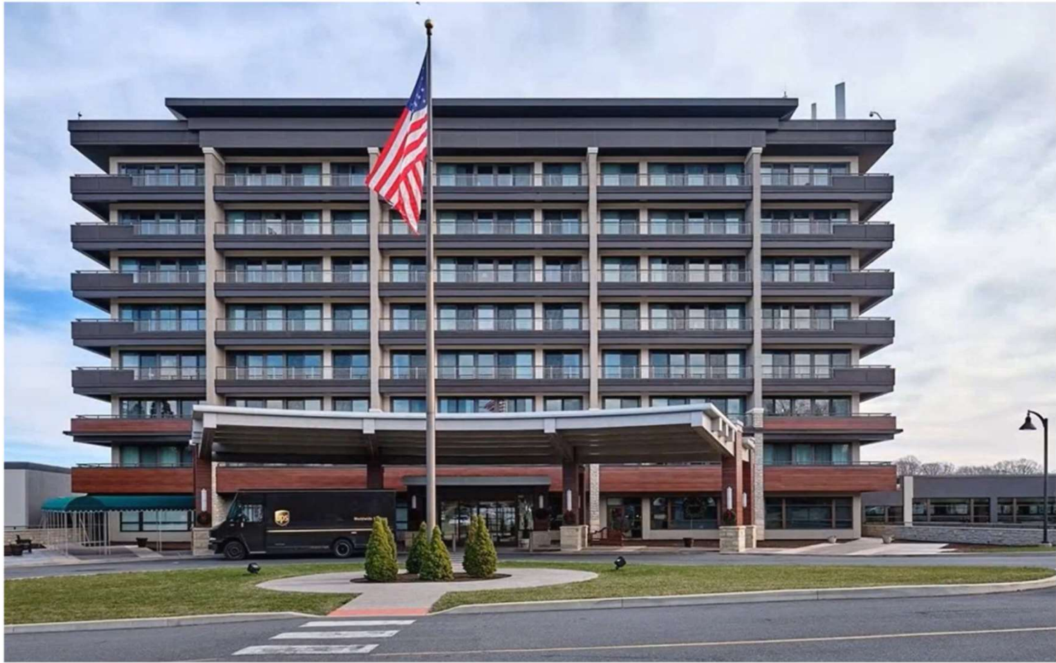
Highrise Community in Hockessin, Delaware (Cokesbury Village)
